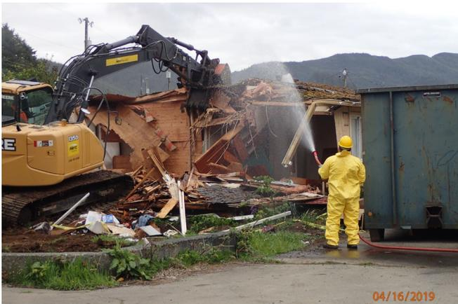
**A remediation contractor applies water to demolition work at the Family Housing Area to limit hazardous dust exposure.**
